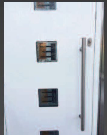
Internal view of door
